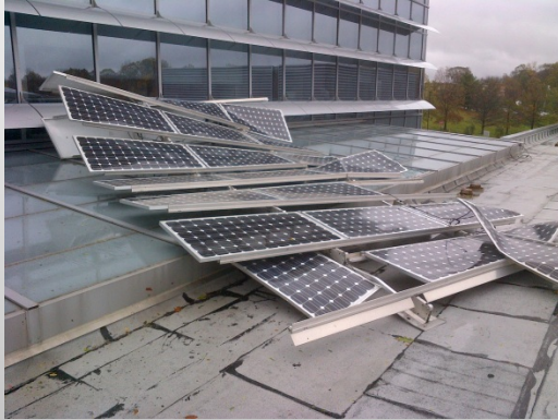
Scott's Lab: Roof view
