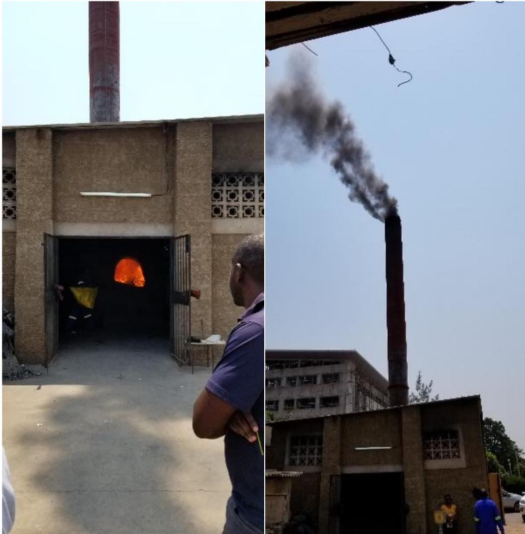
2-Arthur DH: The photo at ADH shows a non-functional Macroburn Unit. This project plans to replace the non-functional unit with a 70kg Unit. The housing, especially the roof, will need to be worked on before installation of new unit.
