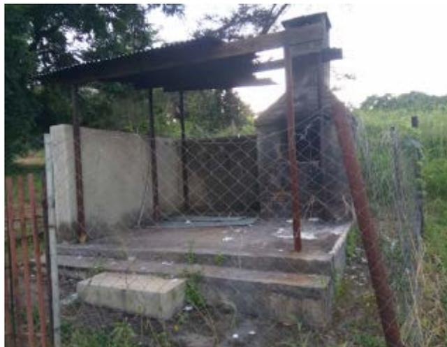
At Choma General Hospital there is only a concrete slab and a partially completed wall plus an incomplete roof. The housing and roof must be completed before installation of new 70 kg incinerator.
